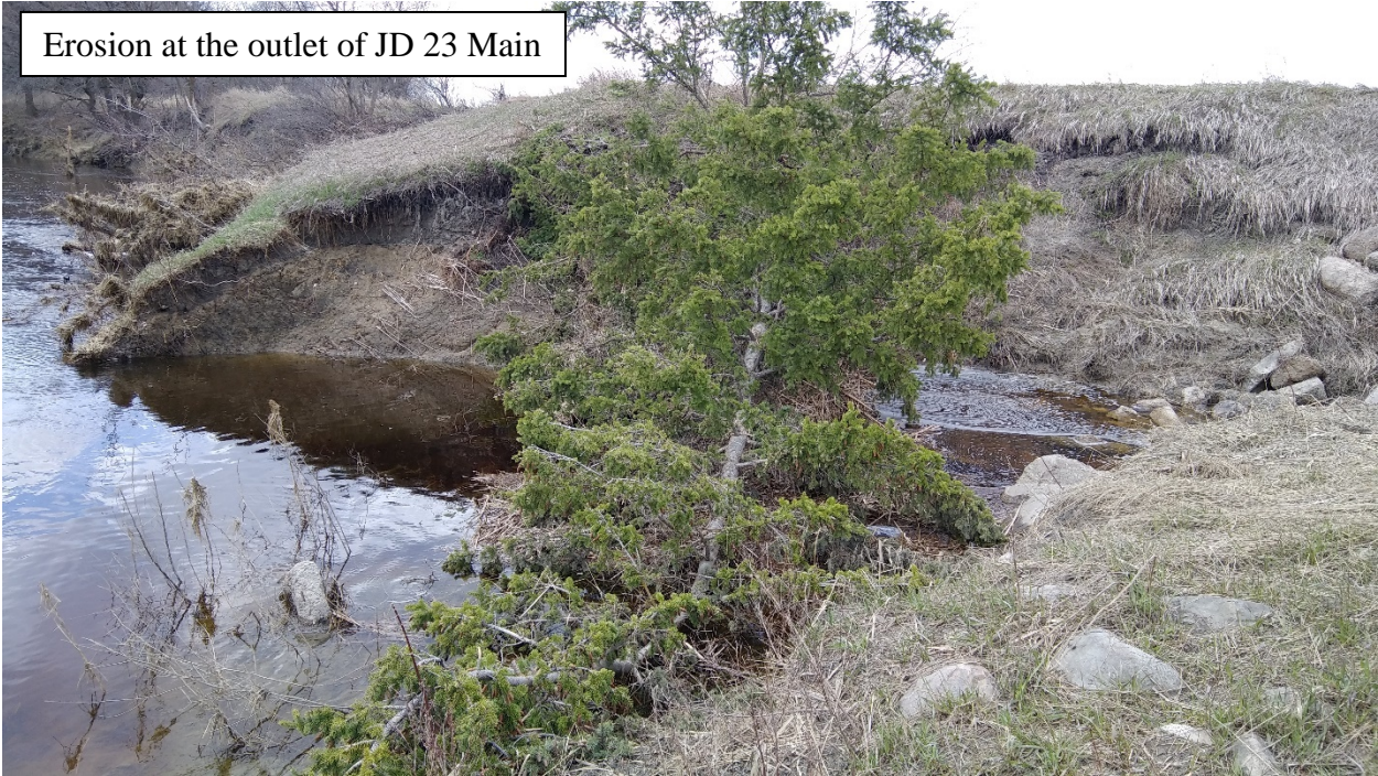
Bank failures along 140 th Ave NE, near the outlet of JD 23 Main
