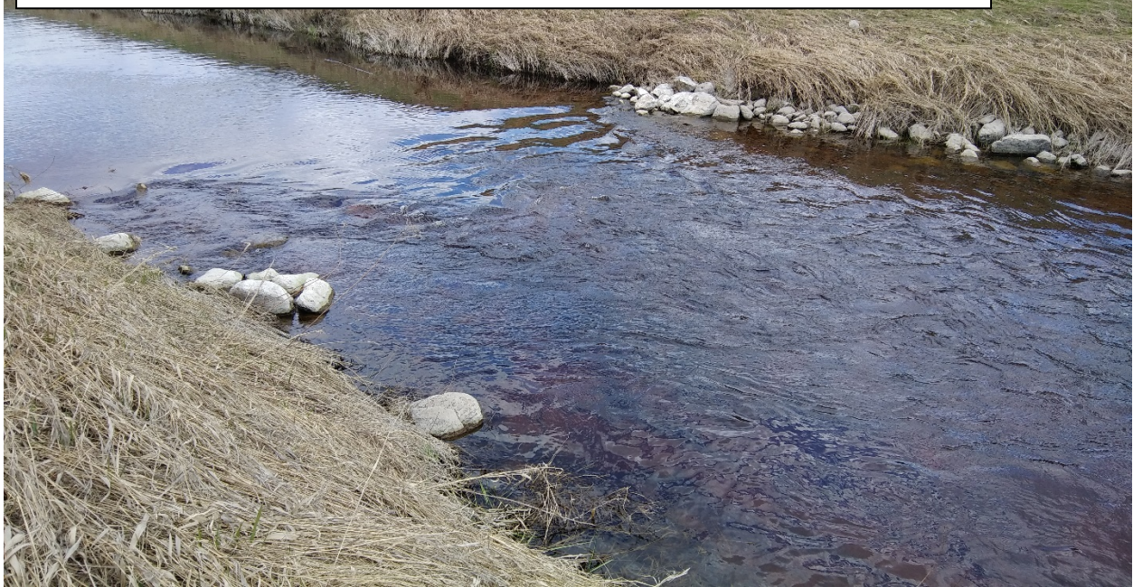
Rock riffle grade stabilization structure in Marshall County Ditch 20 – still working well
